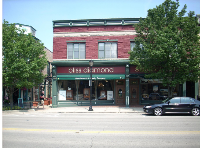
Photo Id: 512-514N Milwaukee Ave
